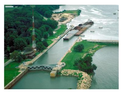
concrete in 1982. The 52-foot-long ice chute section of the dam includes a 52-foot-long inoperable Tainter gate. The lock is the standard 600 feet long by 110 feet wide. The maximum lift is 18.5 feet with an average lift of 17 feet. It takes approximately 12 minutes to fill the lock chamber; nine minutes to empty.
