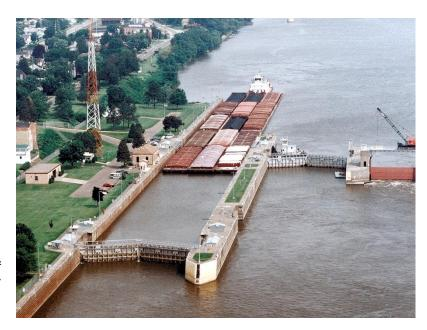
Lock dimensions are 110 feet wide by 600 feet long with additional provisions for an auxiliary lock. The maximum lift is 9 feet with an average lift of 6 feet. It takes approximately 10 minutes to fill or empty the lock chamber.
