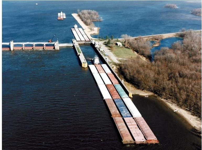
The movable dam consists of 10 submersible Tainter gates, 20-feet high by 64-feet long; and three submersible roller gates, 20-feet high by 100-feet long. The dam system also includes three non-overflow earth and sand-filled dikes; two transitional dikes; and a submersible earth and sand-filled dike. It takes 10 hours for water to travel from Lock and Dam 12, in Bellevue, Iowa, to Lock and Dam 13.
