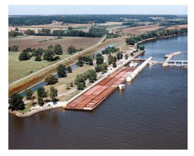
The movable dam has three non-submersible roller gates (20 feet high by 60 feet long), 34 non-submersible Tainter gates (20 feet high by 40 feet long), and six submersible Tainter gates (20 feet high by 40 feet long). The submersible Tainter gates submerge three feet. It takes six hours for water to travel from Lock and Dam 19, in Keokuk, Iowa, to Lock and Dam 20.
