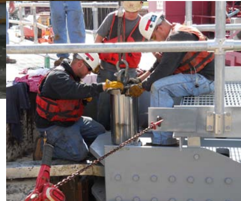
Above, an old gate is mitered with a new gate following its successful installation by the Mississippi River Project Structures Maintenance Unit at Lock and Dam 20 in October. Right, Dan Guise (left) and Justin Carter help guide the pin being lifted by the Liebherr Crane into place securing the miter gate to the lock wall. Also in the photograph is Tim Scranton. Photos by Eric Johnson.
