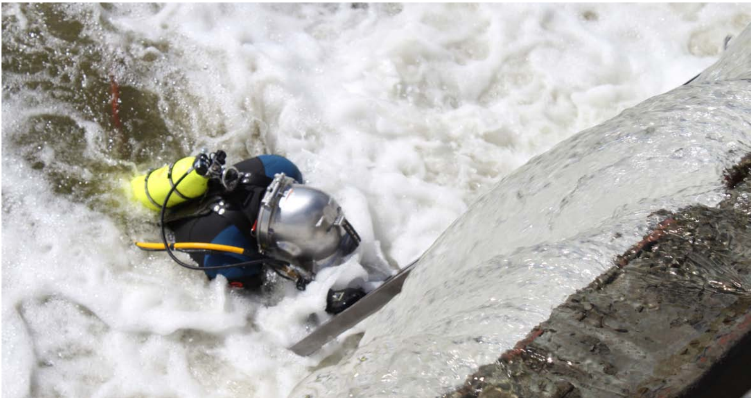
John Snell, diver and lock and dam operator at Starved Rock, begins his submersion to pull bearings on the wicket dam in preparation for dewatering operations.
