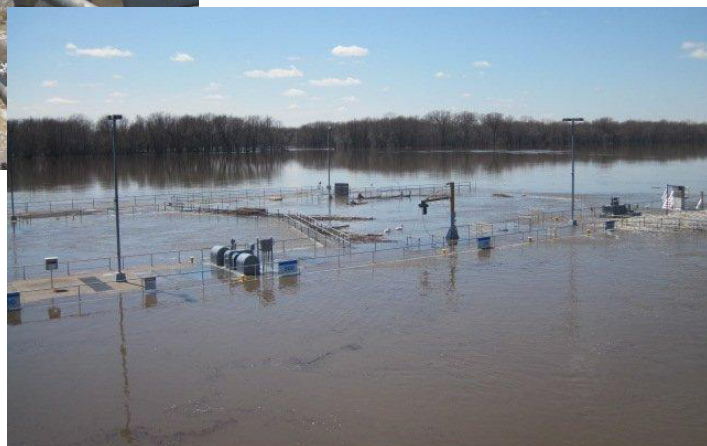
Below, flood waters overtop the lock gates and the wall at Lock 17 April 20. Photo by Bill Ford
