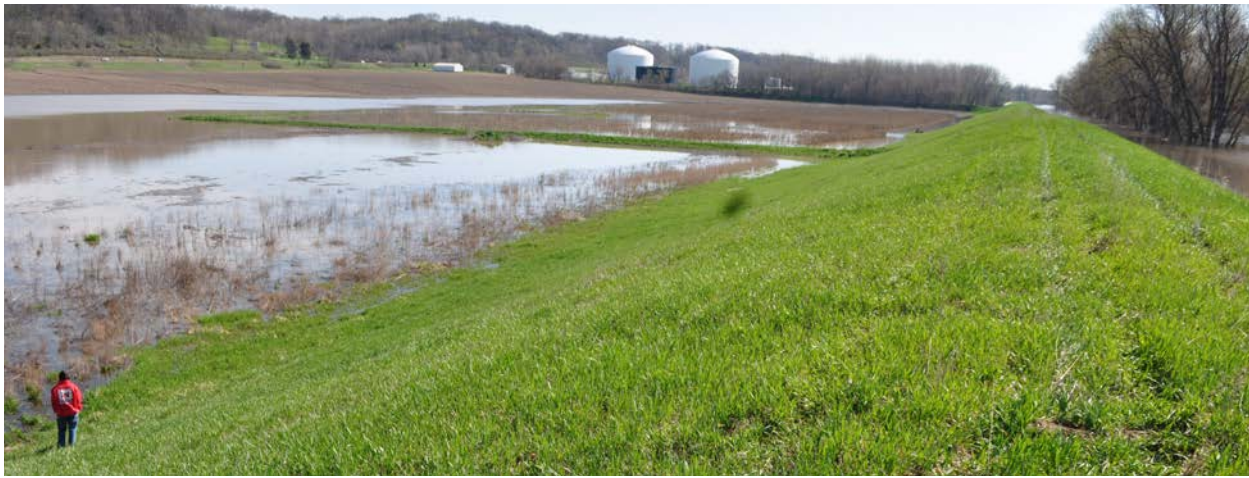
Flood Area Engineer Felix Castro inspects the landside toe of the Banner Drainage and Levee District levee for possible seepage from the Illinois River April 22. Photo by Anthony Heddlesten
