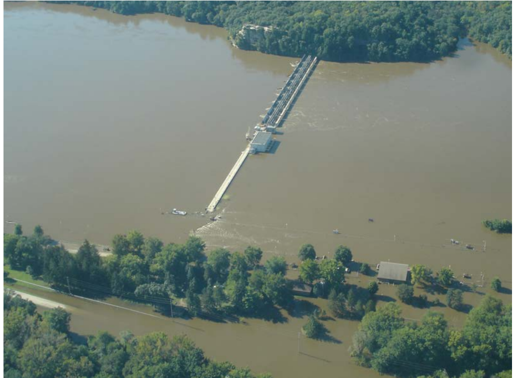
Record setting flood waters on the Illinois River in April inundated Starved Rock Lock and Dam and the adjoining Illinois Waterway Visitor Center. Photo by Illinois Waterway Project Staff
