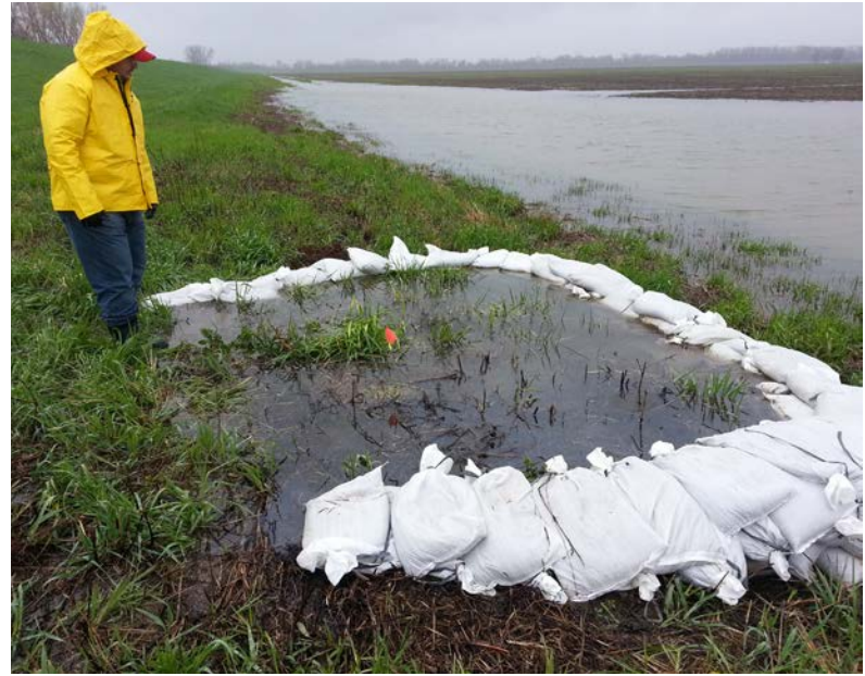
Bryan Snook, Flood Area Engineer assistant, inspects a boil at Indian Graves Upper. Photo by John Hayes
