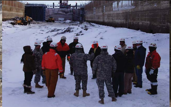
During the two month dewatering project, the work crew had 47 days where temperatures never climbed above freezing. Courtesy Photo
