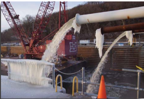
Four, 12-inch pumps were used to to dewater the chamber at Lock and Dam 22. Photo by Aaron Dunlop
