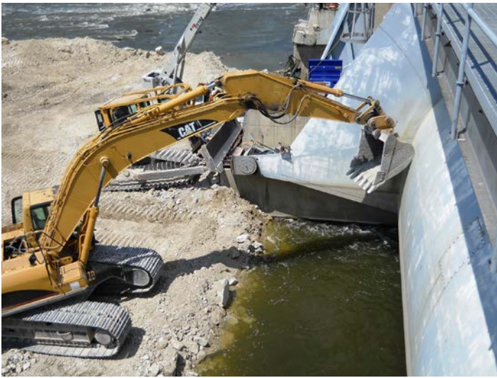
An excavator pushes on Gate 2 at the Marseilles Dam to reposition the gate so the temporary trunnion anchorage can be installed. Photo by Kirk Atwater
