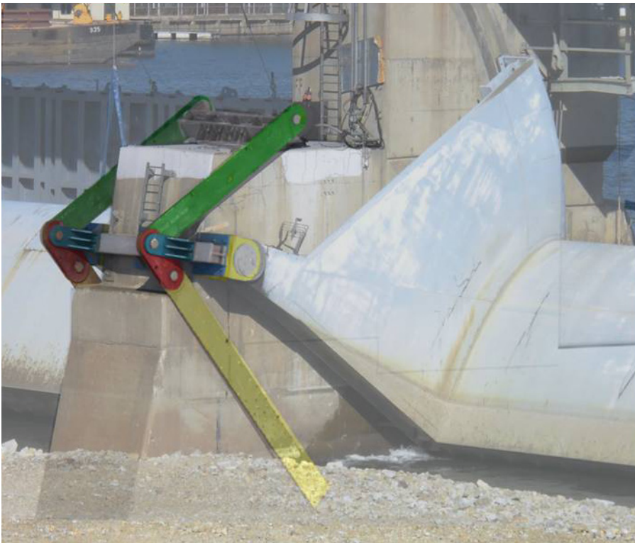
An image of the design for the temporary trunnion anchorage for Pier 2 of the Marseilles Dam is laid over top of what was installed in July. Gates 2 and 3 were successfully attached to the temporary trunnion anchorage, which serves as a pivot point for the gates as they are moved up and down to maintain the 9-foot navigation channel on the Illinois River. The gates and the trunnion anchorage were damaged when a tow moving barges on the Illinois River lost control April 18 in the strong river currents and ended up against the dam. Photo by Kirk Atwater
