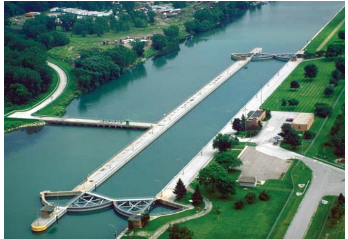
The T.J. O'Brien Lock in Chicago, Ill., is scheduled for repairs this winter and will be closed for navigation during two separate closures. Rock Island District photo
