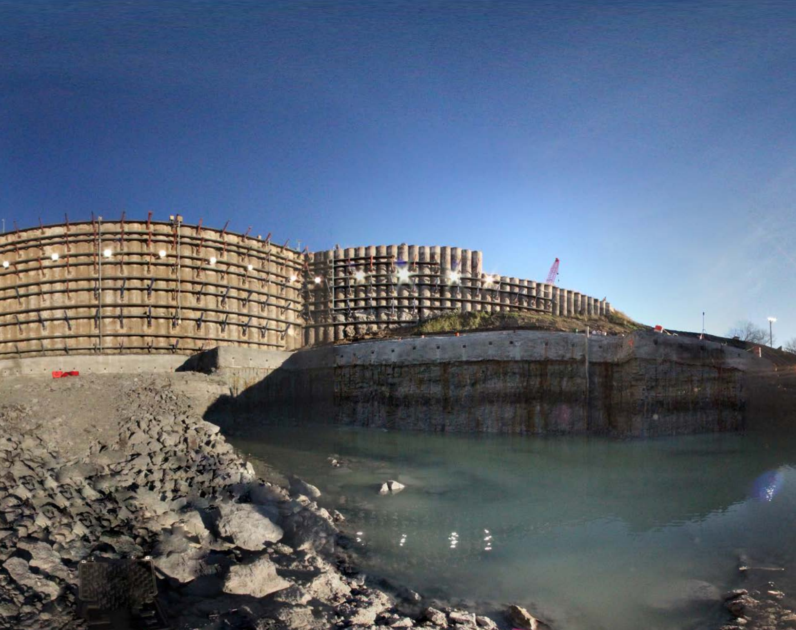
A 360-degree view of the construction area below Lake Red Rock Dam where construction is ongoing for a hydroelectric powerhouse. The large wall in the center of the image is a secant pile wall, designed to keep the earthen dam stable during excavation and construction. The large rocks at the bottom of the image are a result of blasting efforts by the contractor to remove the final layers of bedrock from the area where the powerhouse foundation will be set. Photo by Joss Voss (enhanced for publication)
