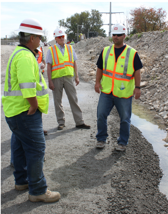
Geotechnical engineer, Eric Hackbarth (right), explains the benefits of using roller-compacted concrete for the Lockport forebay wall to safety specialist, Jim Trail (left), and cost engineering specialist Chuck Van Laarhoven (center). Photo by Samantha Heilig
