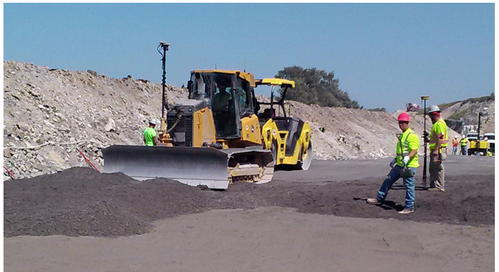
Contractors working on the new forebay wall at the Lockport Lock and Dam Upper Pool project use a bulldozer to spread a mixture of cement, water and crushed rock used in creating roller-compacted concrete (RCC). In total, the wall will contain approximately 80,000 cubic yards of RCC and will take nearly 4,000 off-road dump trucks to place the material. Photo by Eric Hackbarth
