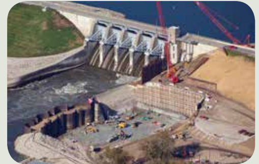
The District authorized use of the Lake Red Rock Dam for construction of a hydroelectric power plant with a completion date in 2018.
