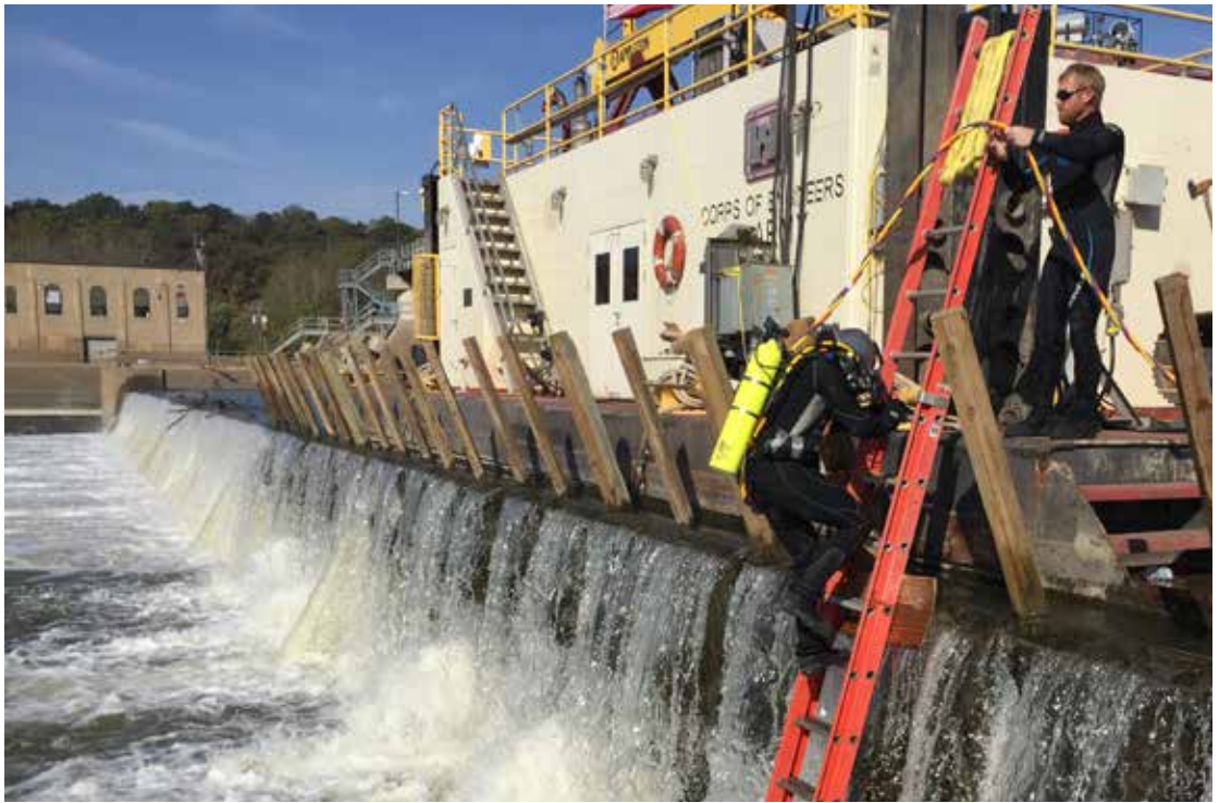
Diver, Brandon Hornung, enters the water below the dam at LaGrange Lock and Dam, assisted by tender Curtis Brown. Hornung works as Assistant Lockmaster at Starved Rock Lock and Dam but he also works as a member of the District's dive team.
