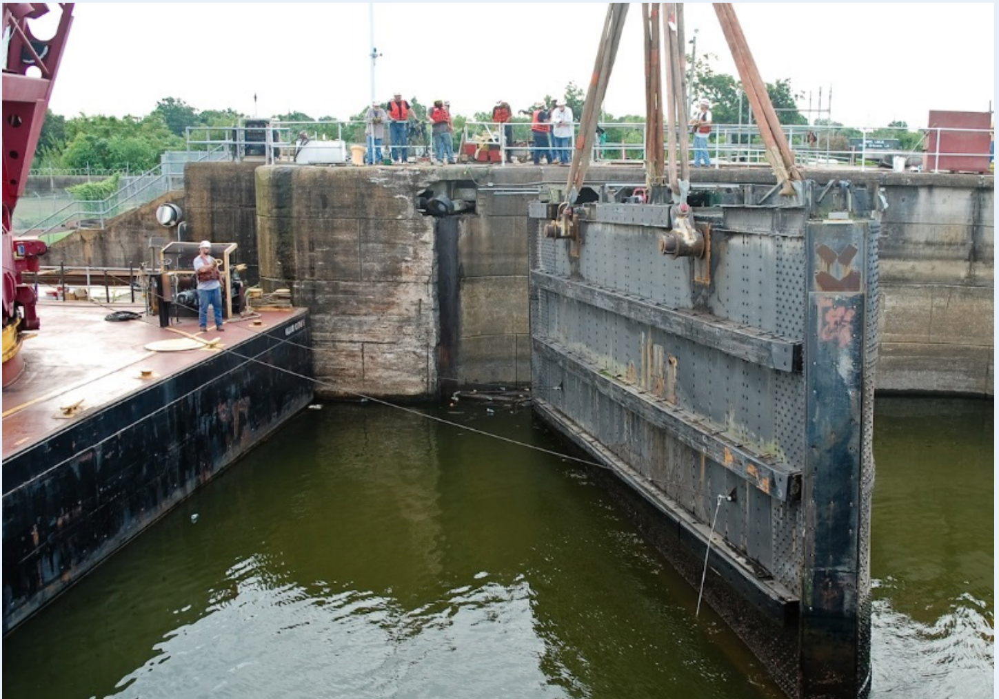
Maintenance crews from Rock Island and New Orleans Districts use the Quad Cities Lift Crane to remove the No. 8 gate from the Inland Harbor Navigational Canal (IHNC) Lock in New Orleans.
