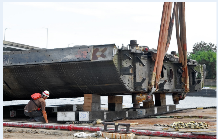
A maintenance crew member watches closely as the Quad Cities Lift Crane slowly lowers the IHNC lock gate onto supports that will hold the gate in place as it is moved. Photo provided by Justin Carter
