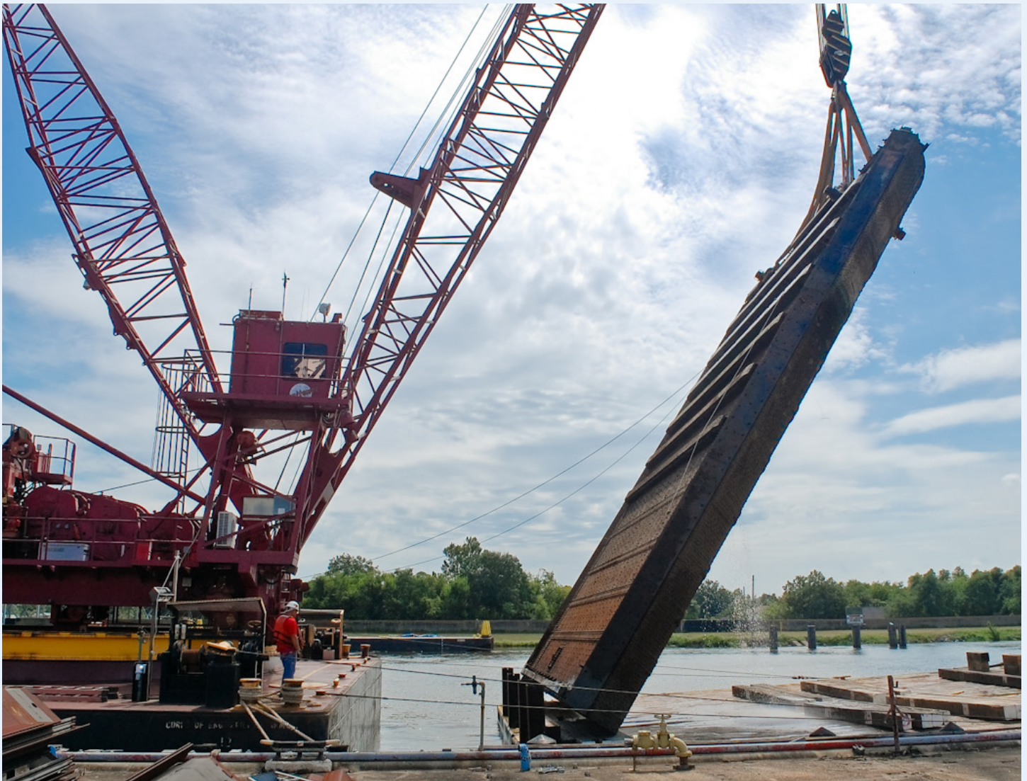
The Quad Cities Lift Crane carefully lowers a 574,000 pound IHNC Lock gate onto the work barge of the Motor Vessel Bettendorf during a dewatering project in News Orleans, Louisiana. Photo provided by Justin Carter
