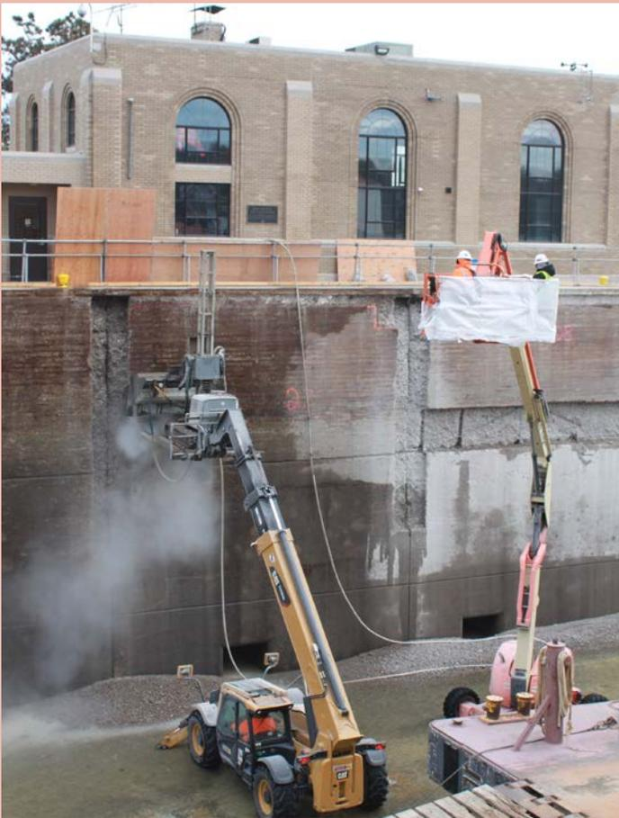
**A hydro-demolition machine was used at Lock 17 to remove old concrete from the lock walls. Photo by Samantha Heilig**
