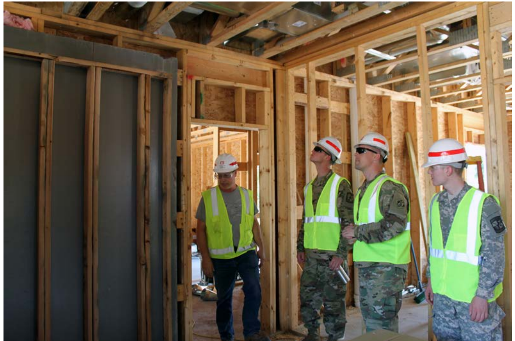
Louisville District Project Engineer Gerald Zerphey, far left, explains the importance of the reinforced metal between the studs during a site tour for the District’s visiting cadets. Each home is equipped with a safe room to help protect residents during bad weather. Photo by Katherine Rosario
