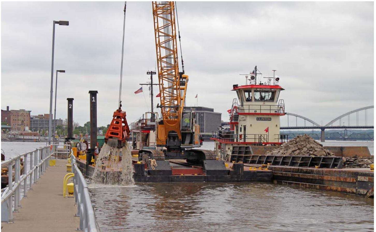
Mississippi River Project maintenance crews with the U.S. Army Corps of Engineers, Rock Island District, demolish a portion of the lower guidewall at Locks and Dam 15 in Rock Island, Illinois. Removing the concrete will prevent the wall from falling into the river in an uncontrolled manner. Photo by Katherine Rosario
