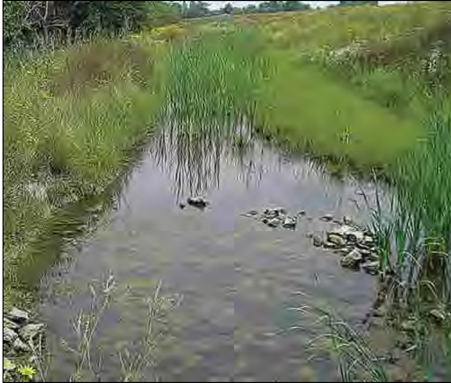
Photograph 4-4. Sediment Retention Structure
