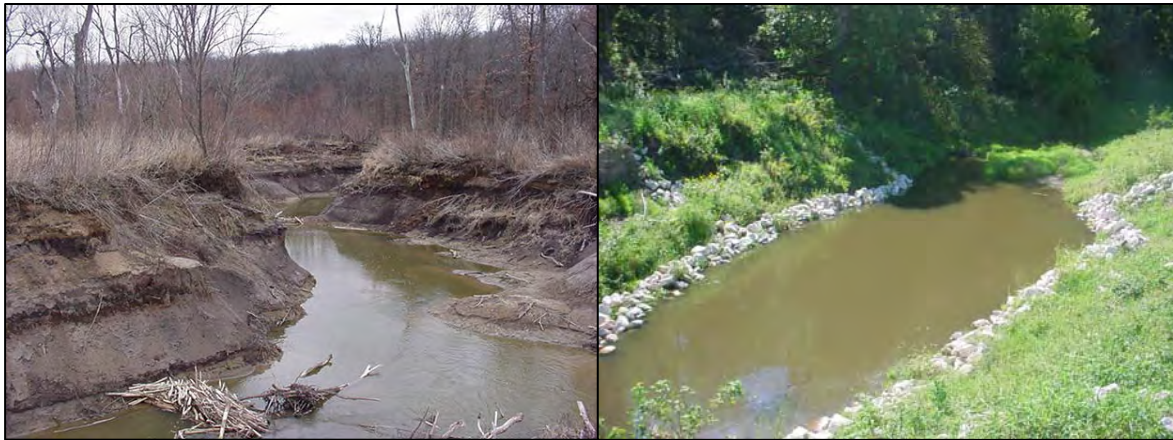
Photograph ES-1. Example before and after stream restoration with stone toe protection
