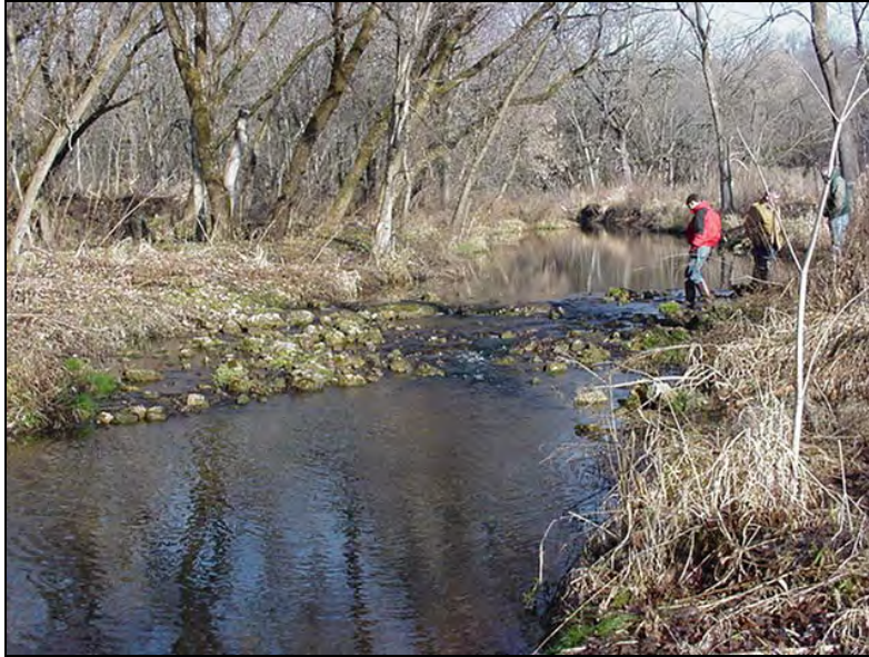
Photograph 4-1. Riffle Structure for Grade Stabilization
