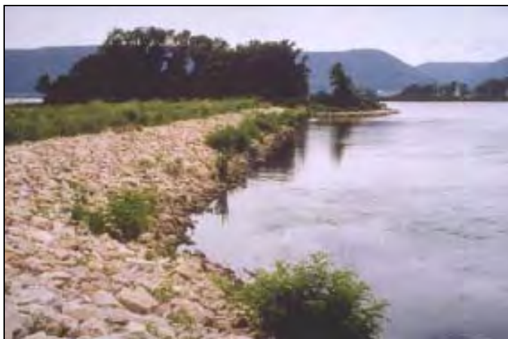
Photograph 4-2. Rock Revetment Used for Bank Stabilization
