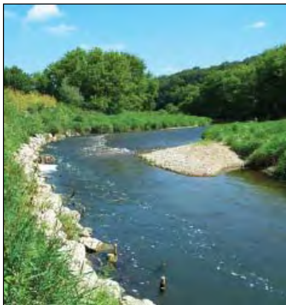
Photograph 4-3. Bioengineered Stone Toe Protection and Vegetation Used for Bank Stabilization (Univ. of Illinois- Urbana Champaign Water Quality Department: www.wq.uiuc.edu/Pubs/Streambank.pdf )
