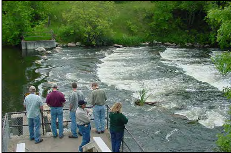
Photograph 3-5. Rock Ramp- Otter Tail River, Minnesota
