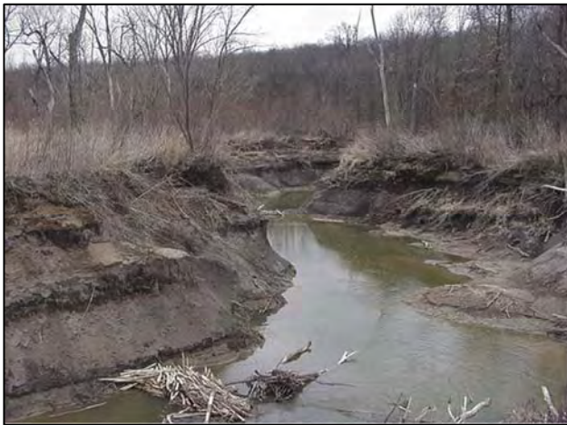
Photograph 2-9. Stream Incision and Stream Bank Erosion
