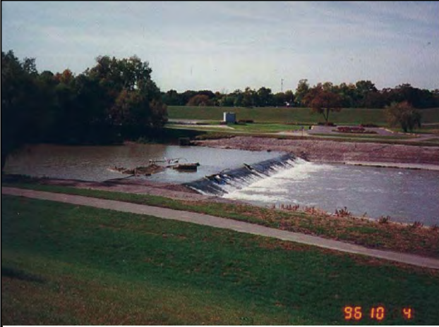
Photograph 2-10. Low Head Dam
