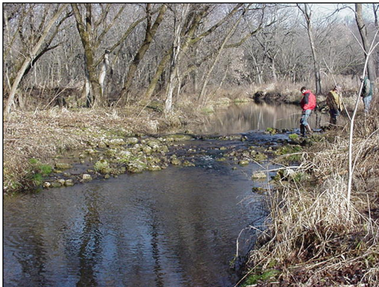
Photograph 4-1. Riffle Structure for Grade Stabilization
