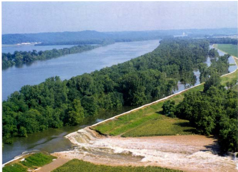
Figure 2.2: Levee Breach (North Central Division, 1994).
