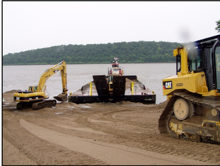
Photograph 2. Typical Mechanical Dredging Offload
