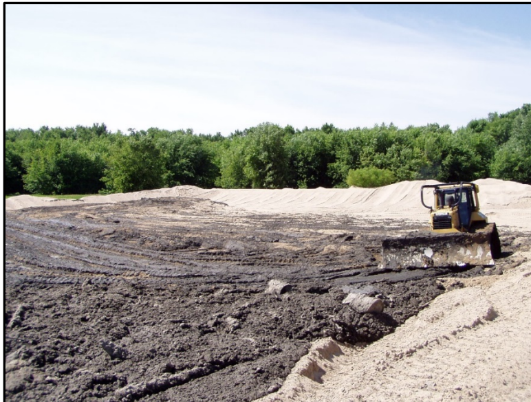
Photograph 3. Mechanical Placement of Fine Materials With Sand Berms at the Edges to Contain the Fines While They Decant
