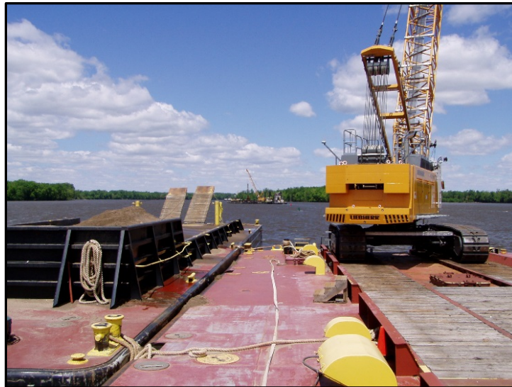
Photograph 1. Mechanical Dredge Placing Material on Deck Barge
