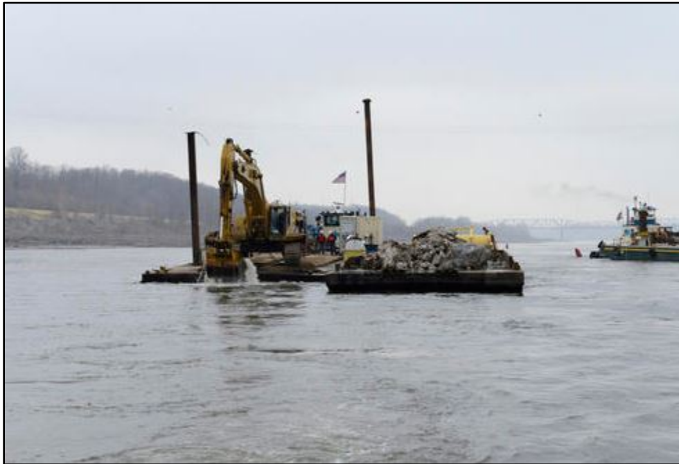
Photograph G-1-9. Mechanical Dredging
