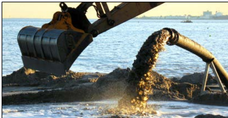
Photograph G-1-8. Hydraulic Dredge Placement (Photograph From Resource Management Group, Inc.)
