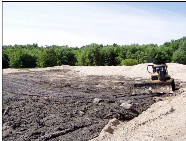
Photograph 6. Mechanical Placement of Fine Materials With Sand Berms at the Edges to Contain the Fines While They Decant
