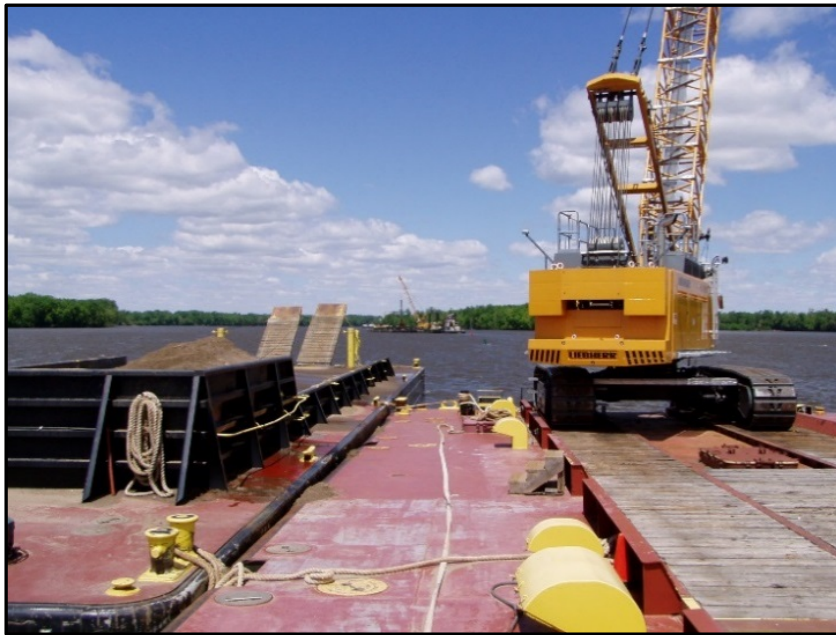
Photograph 4. Mechanical Dredge Placing Material on Deck Barge
