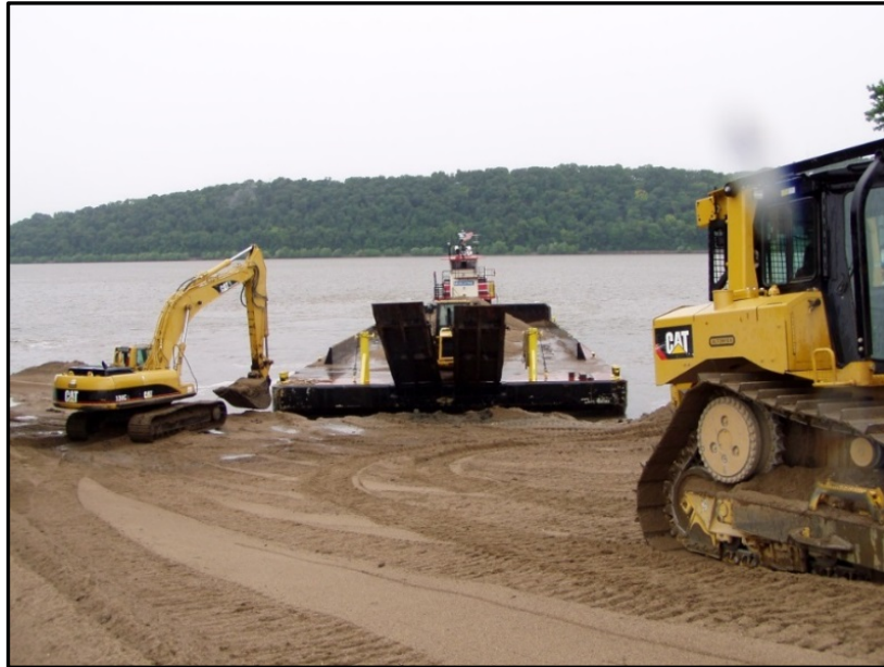
Photograph 5. Typical Mechanical Dredging Offload
