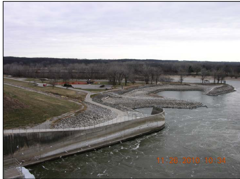
Rip Rap Work in Tailwater
