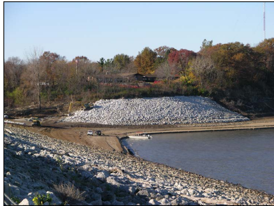
Rip Rap Work at Visitor Center in 2010
