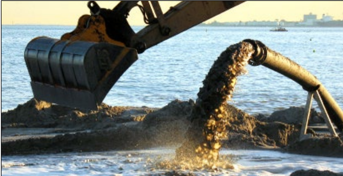
Photograph EA-B-2: Hydraulic Dredge Placement (Photograph from Resource Management Group, Inc.)
