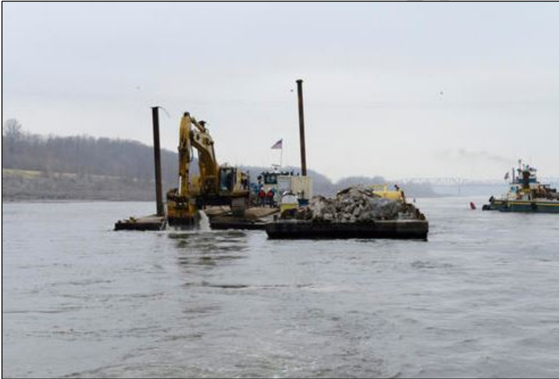
Photograph EA-B-1: Mechanical Dredging
