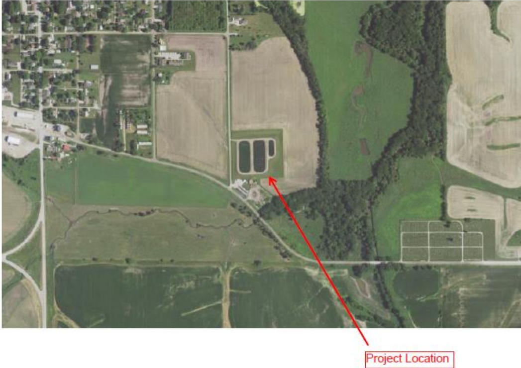
City of Winfield Sewer Improvements Project
