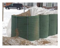
**HESCO Bastion.** The barrier is made of a collapsible wire mesh container and heavy duty fabric liner, and is used as a temporary to semi-permanent dike or
