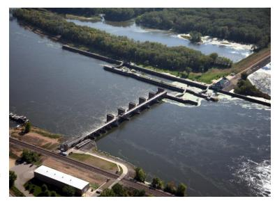
the lock chamber. A partial auxiliary lock consists of an upstream set of miter gates and a short concrete riverwall.
