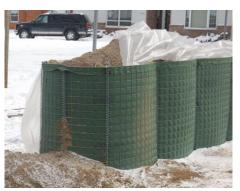
**HESCO Bastion.** The barrier is made of a collapsible wire mesh container and heavy duty fabric liner, and is used as a temporary to semi-permanent dike or
