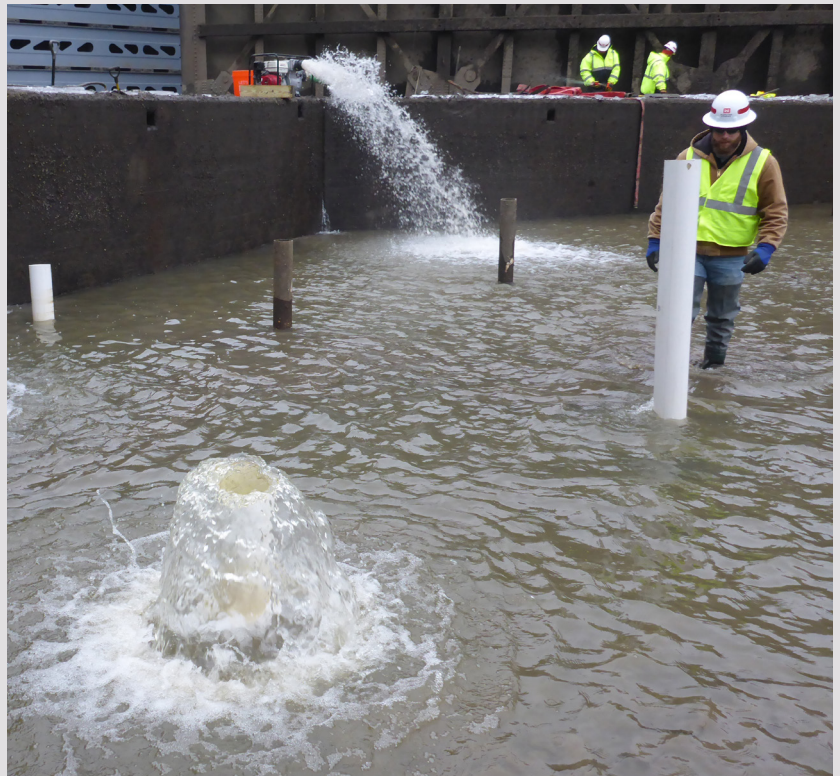
Civil Engineer, Stefan Flynn, inspects the stand-pipes that were installed in the floor of Lock and Dam 13 during the winter dewatering project. These pipes reduced the flow of water and eroded soil entering the chamber through weep holes in the concrete floor. Photo by James Maher
