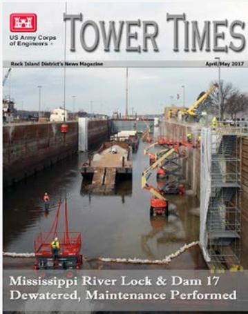
Maintenance crews at Lock and Dam 17, near New Boston, Illinois, perform winter maintenance inside the dewatered lock chamber. *Photo by Samantha Heilig*
