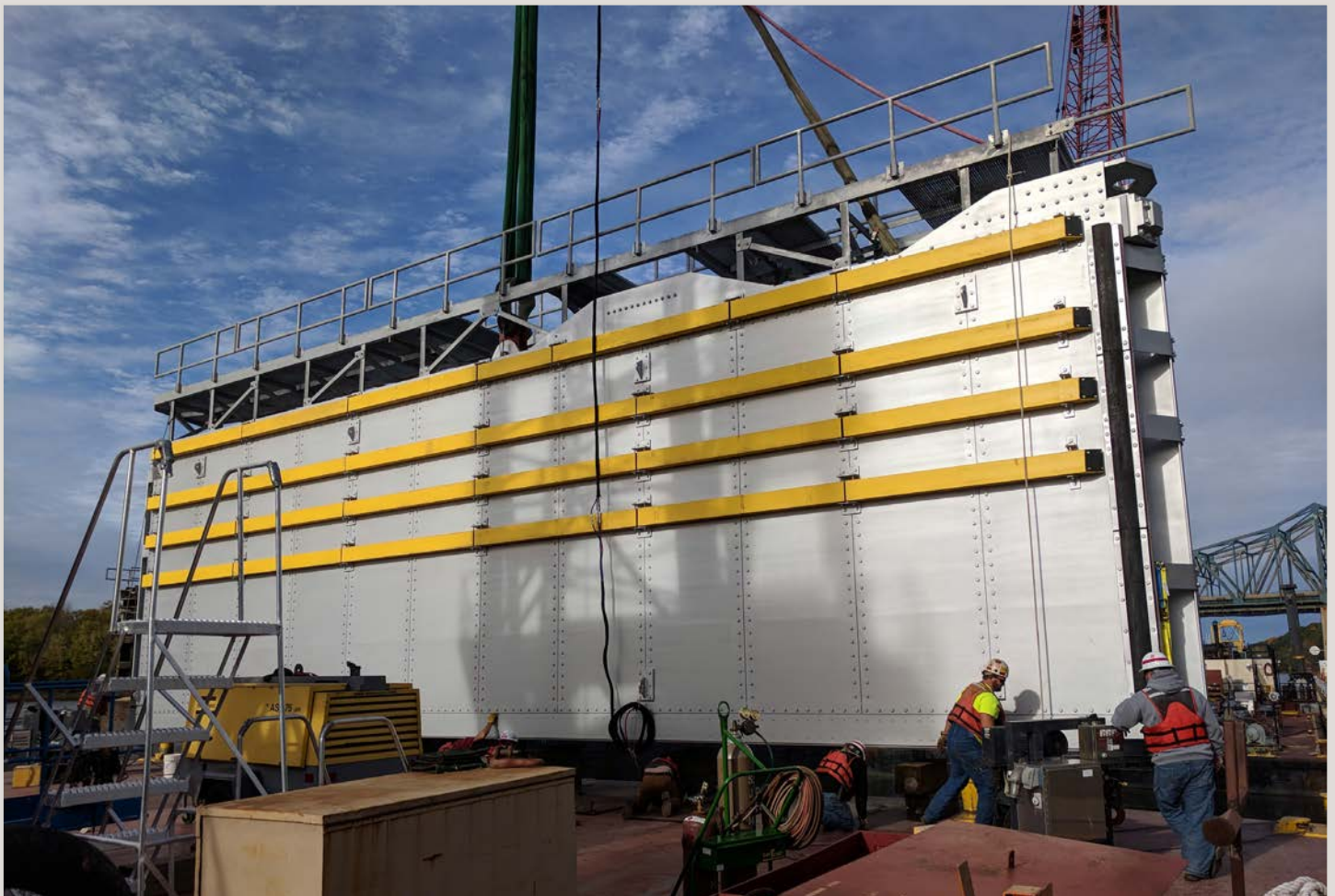
Rock Island District maintenance crews on the Illinois Waterway prepare a newly manufactured miter gate for installation at Peoria Lock. Photo by Doug Morgan
