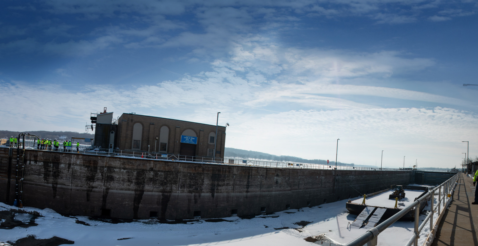
Members of the Quad Cities Riverfront Council, local mayors and members of the local media tour Locks and Dam 14 near LeClaire, Iowa while it was dewatered for winter maintenance. Scaffolding next to lock walls allowed people to walk to the bottom of the river to explore the historic lock. Photo by Kelcy Hanson
