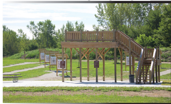
Construction is complete and ready for archers to build their skills on the new archery range at Saylorville Lake.
