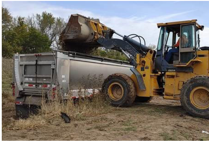
Dredge material from the Illinois Waterway is loaded into a semi trailer to be used in manufactured soil products for commercial sale. Photo provided by Chuck Theiling
