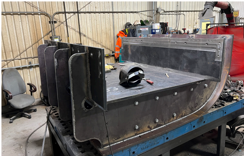
The new rolling feet used for laying miter gates on their side were designed and fabricated in the Rock Island District's maintenance facility at the Mississippi River Project Office in Pleasant Valley, Iowa. Photo by Kirk Atwater
