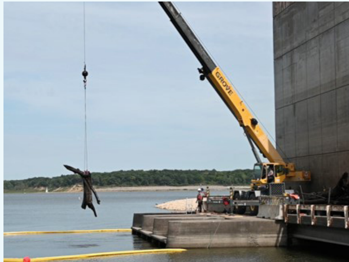
A contractor uses a crane to remove over four decades of debris from the trash rack on the Saylorville Dam control tower. Photo provided by Saylorville Staff
