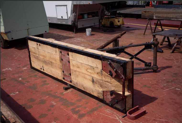
(Top left) Solid oak timbers, used for building wicket gates, lie on a trailer at the Illinois Waterway Project office in Peoria, Illinois, waiting for the next step of assembly. (Bottom left) New wooden wicket assembled and placed on a barge waiting to be transferred to LaGrange Lock and Dam for install. (Right) Tyler Wright, Lock and Dam Repairer, chiseling oak timbers according to blueprints to ensure proper measurements are met before wicket assembly. Photos by Kelcy Hanson
