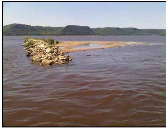
Photograph 9-9. Seed Island With Sand Accumulated on Its Upstream Side
