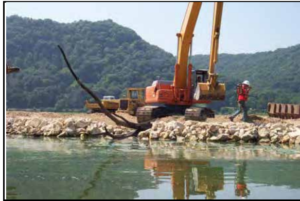
Photograph 9-15. Loafing Structure Being Installed by the Contractor
