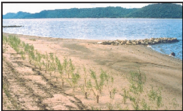
Figure 2-6. Shoreline stabilization features in the Pool 8 Islands Phase II HREP include sacrificial berm material, willow plantings along the beach, and rock groins in the river to deflect currents.
