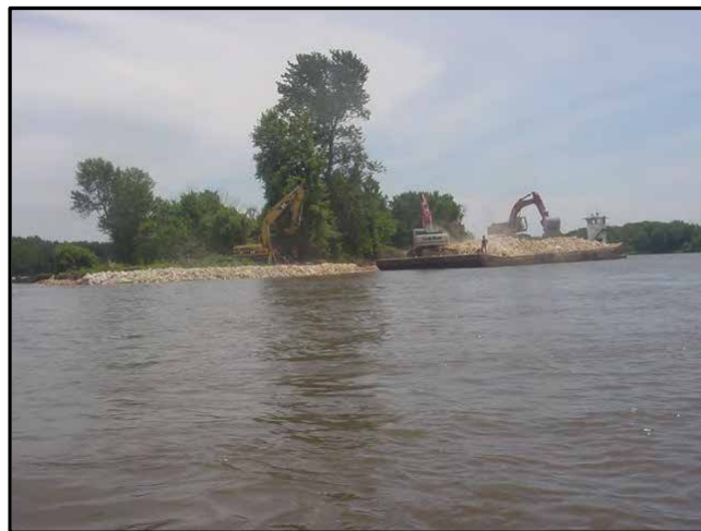
Photograph 4-9. Placement of Rock Revetment at Long Island
