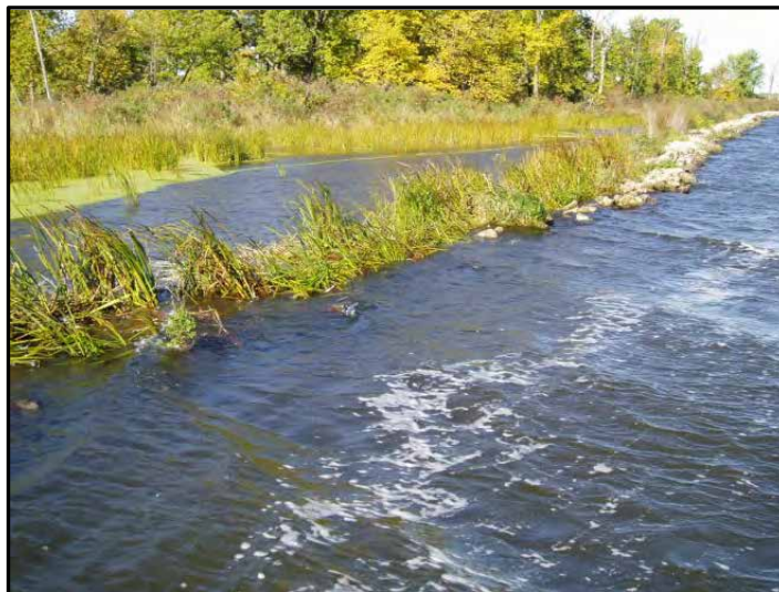
Photograph 4-15. Offshore Rock Mound at Peterson Lake in Pool 4
