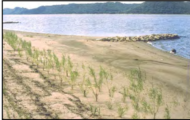
Photograph 4.3. Bio-Geo Stabilization with Groins and Willows (Boomerang Island)
