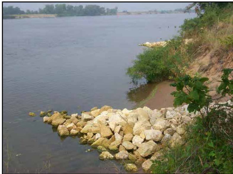
Photograph 4-13. Rock Vanes at Lost Island Chute, Pool 5
