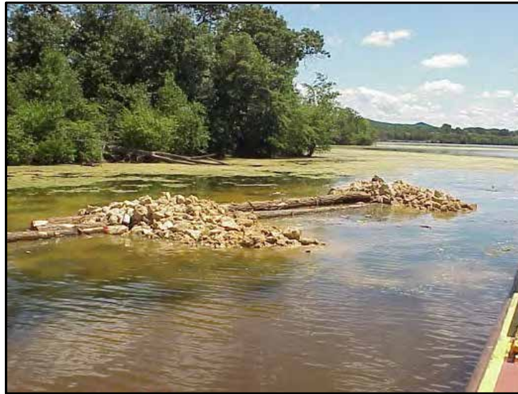
Photograph 4-17. Rock-log Structure in Place
