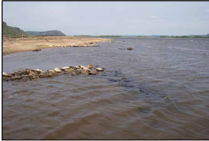
Photograph 4-14. J-Hook Vane in Pool 8
