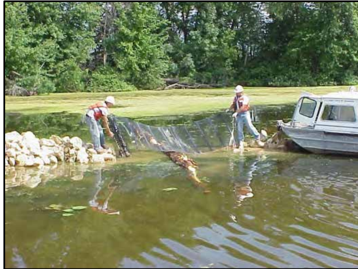
Photograph 4-16. Installation of a Rock log Structure
