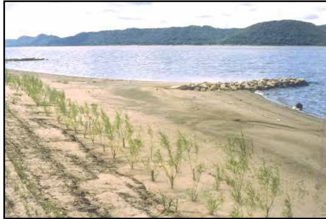
Photograph 4-11. Newly Constructed Rock Groin in Pool 8
