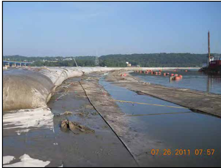
Photograph 6-5. High Solids Geotextile Containers Placement Peoria, IL
