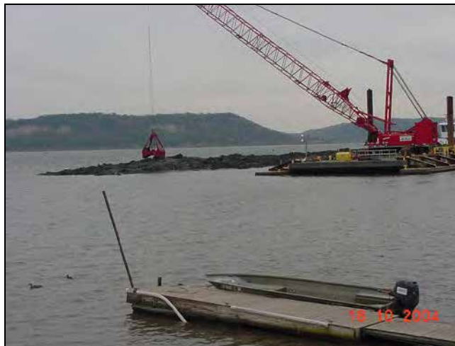
Photograph 6-1. Clamshell Dredge Side Casting Material at Mud Lake, IA
