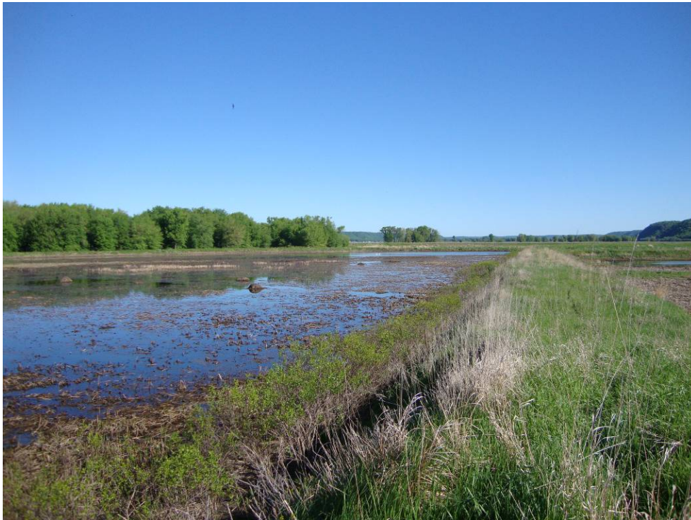
Photo 18: Area 2 southeast corner looking north.
