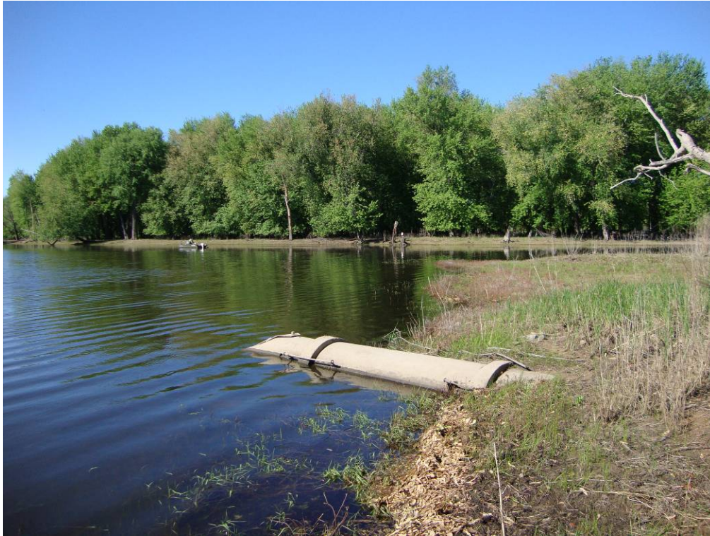
Photo 7: Outlet No. 2 exterior outlet, looking southwest.
