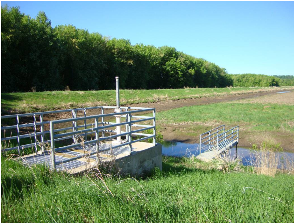
Photo 1: Outlet No. 1 looking southwest. Area 1 dewatered.
