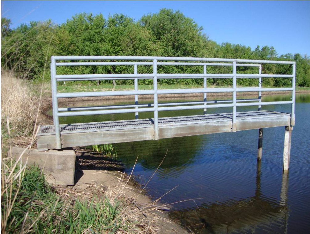
Photo 5: Outlet No. 2 walkway upper footing undermined.
