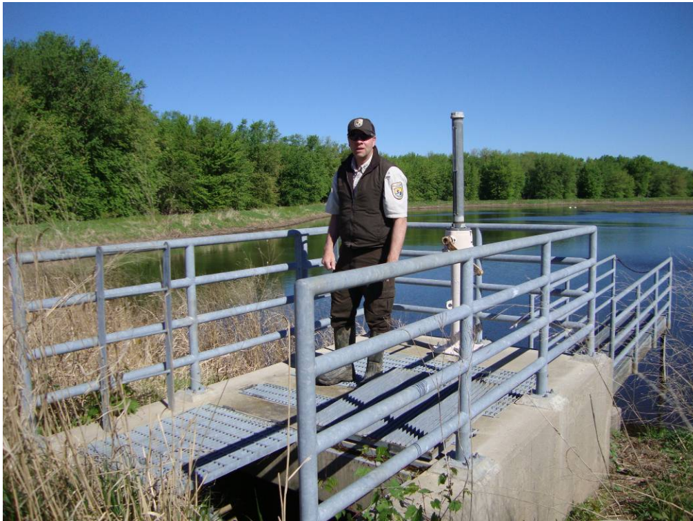
Photo 4: Outlet No. 2 looking northwest. Yager.
