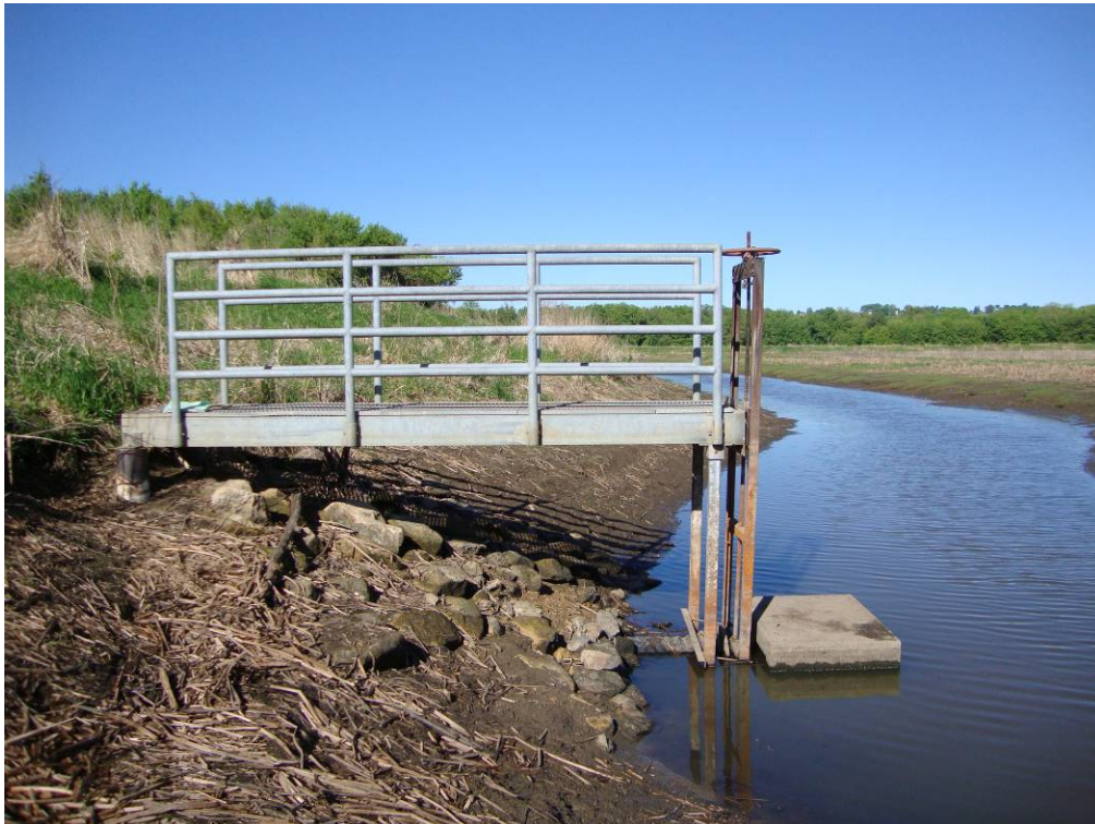
Photo 8: Outlet No. 3, looking west. Area 1 dewatered.
