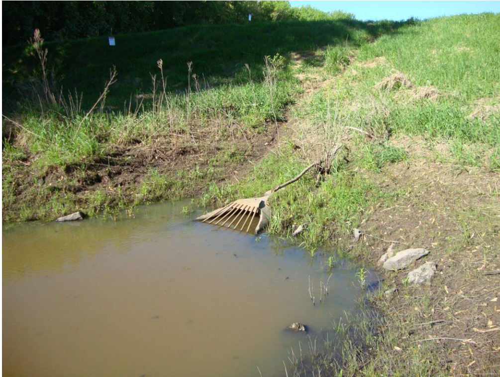
Photo 3: Outlet No. 1, exterior outlet.
