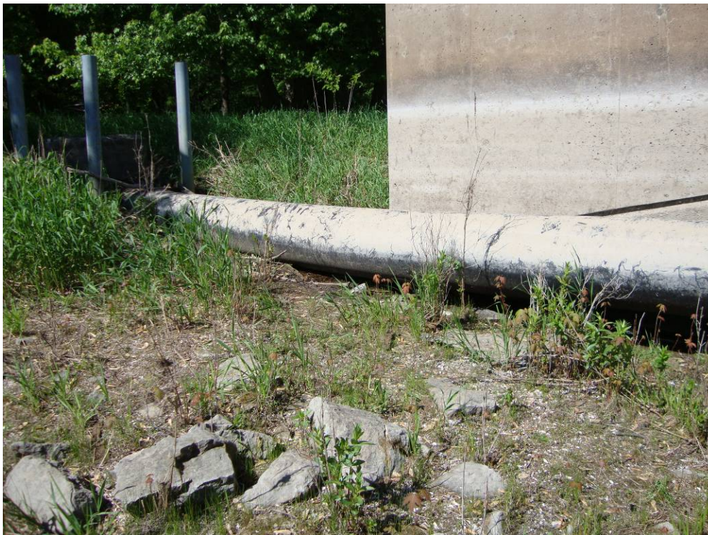
Photo 10: Water supply line looking toward manhole. Losing support underneath this portion of pipe.
