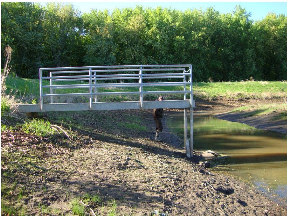
Photo 2: Outlet No. 1 walkway looking south. Area 1 dewatered. Yager behind structure.
