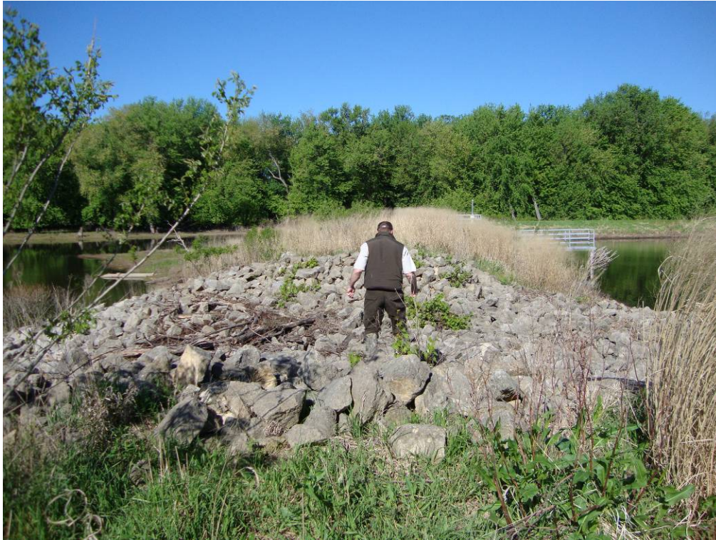
Photo 13: Spillway looking west. Yager.
