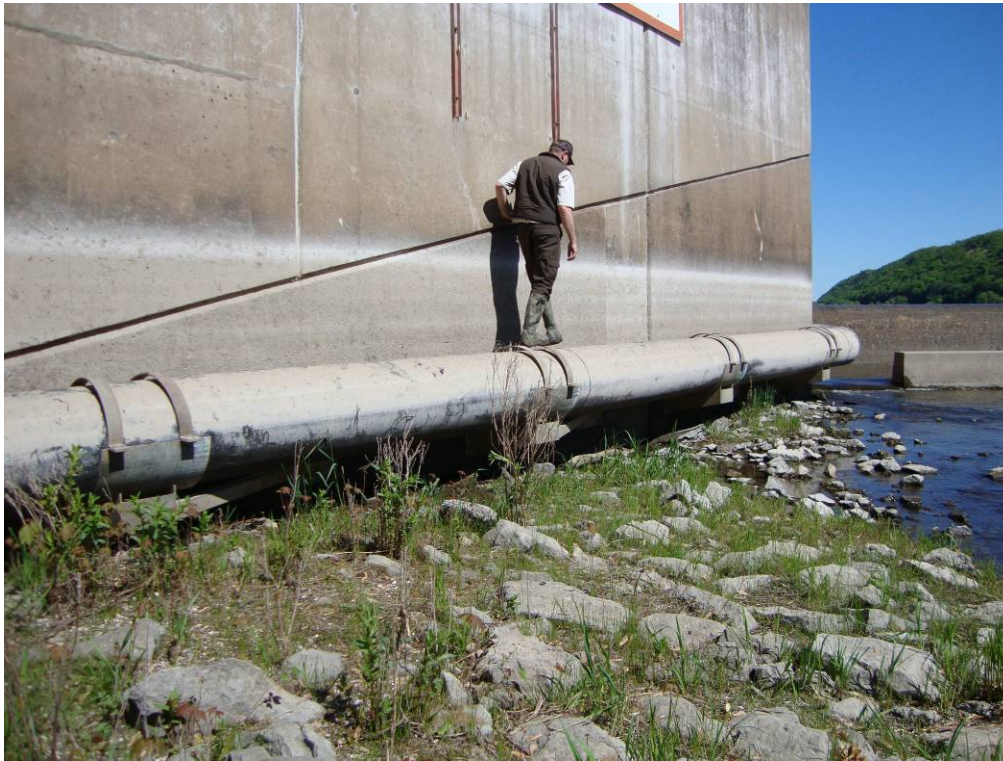
Photo 9: Water supply line along spillway wall, looking towards spillway. Yager walking line.
