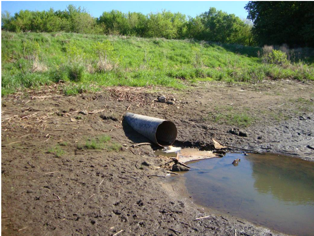
Photo 12: Water supply line, outlet into Area 1. Apron rusted and no longer on end of pipe.
