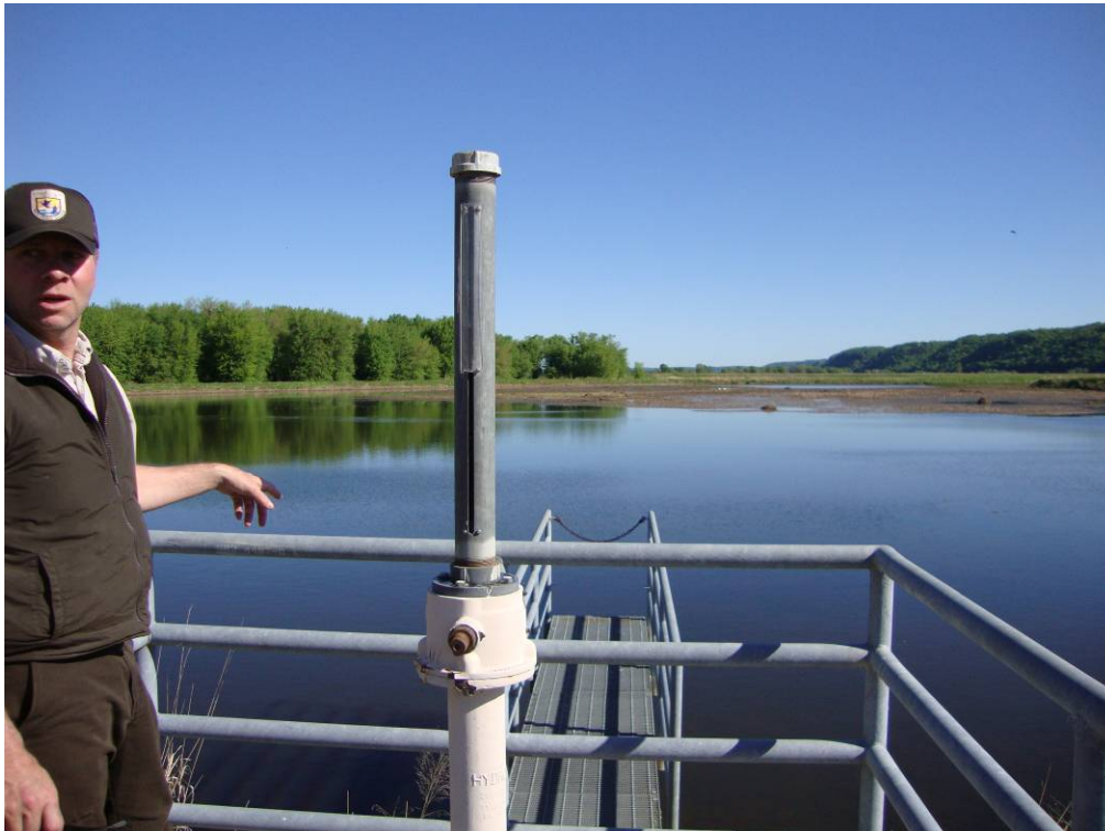
Photo 6: Outlet No. 2 broken Plexiglas on gate well stem cover. Yager.
