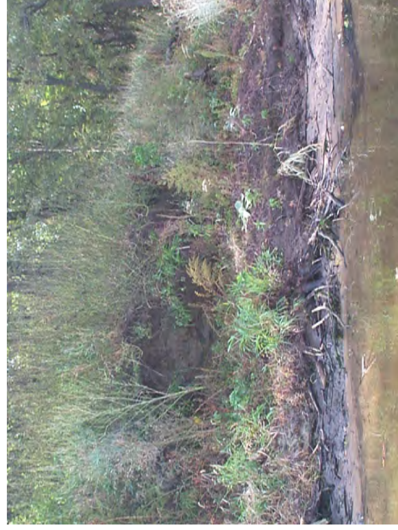
Bank Sloughing at Entrance to Access Channel
