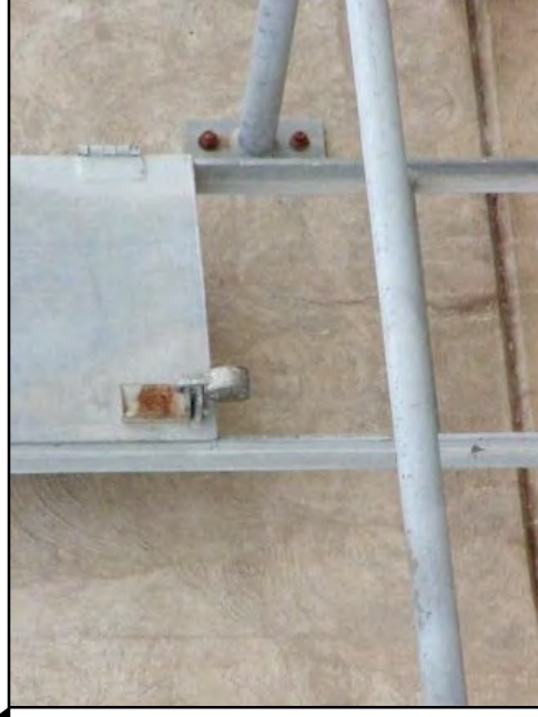
Security measure for the access ladder
