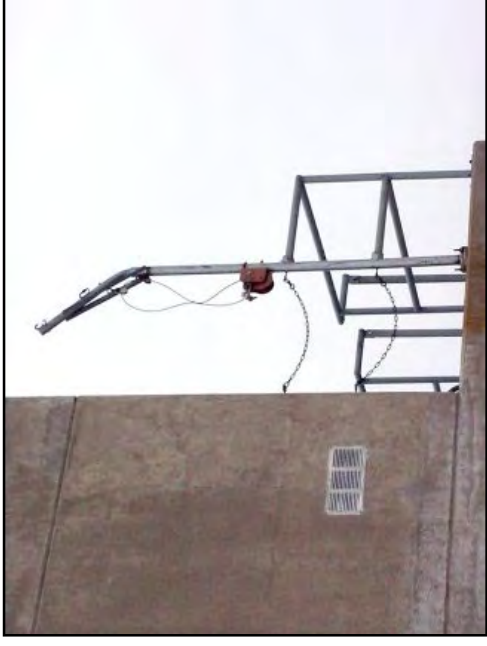
Manual hoist & job crane mounted to handrail
