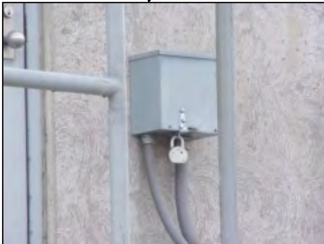
Security measure for the utility box
