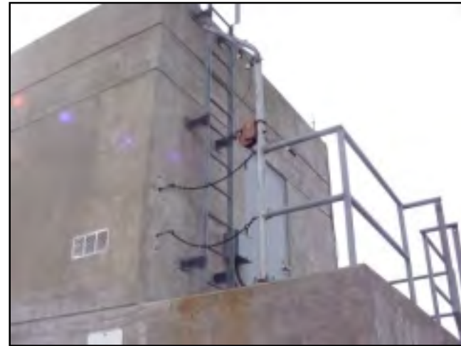
Manual hoist and jib crane mounted to handrail
