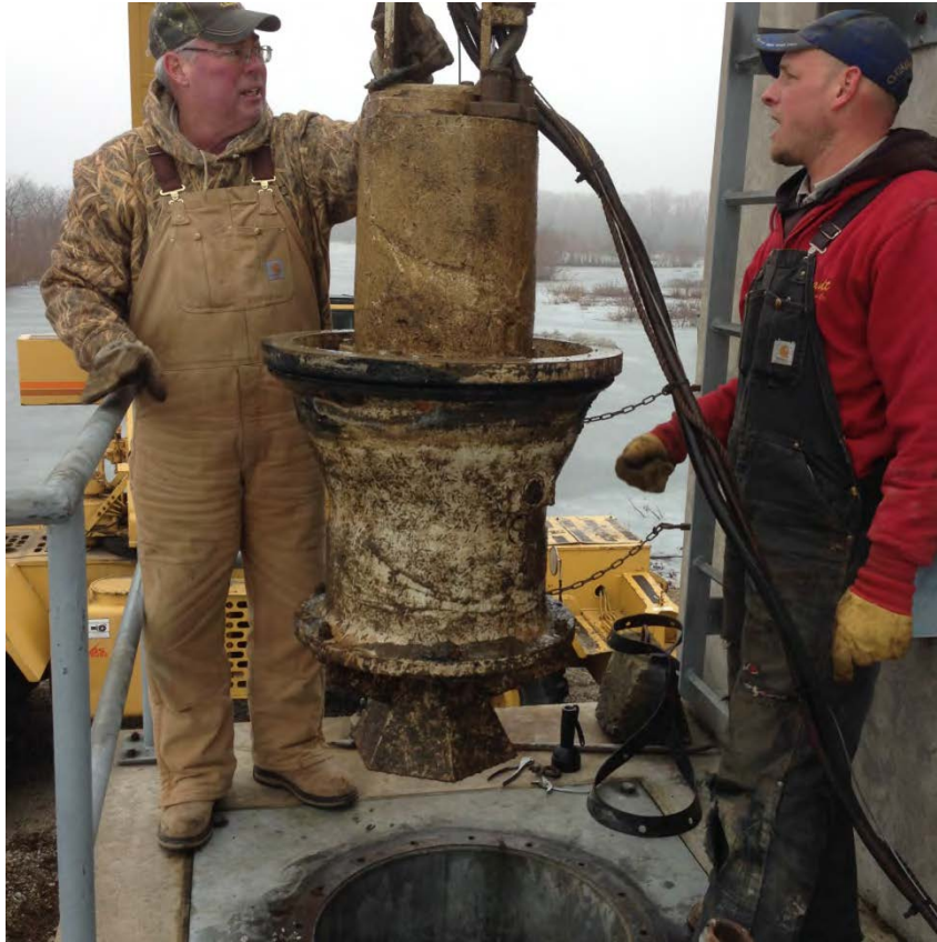
Photo 4: Pumphouse, winter 2016, preparing for pump removal.
