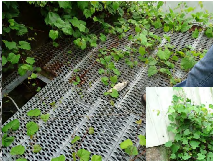
Vegetation encroaching on intake structure
