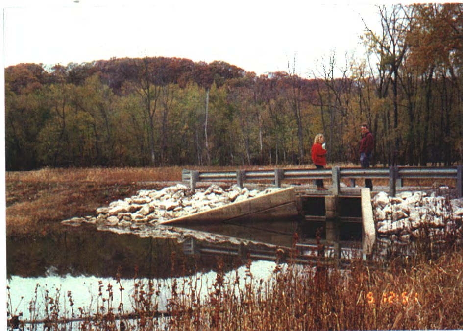
Photo 8. Intermediate (interior) water control structure (2-bay stop logs)
