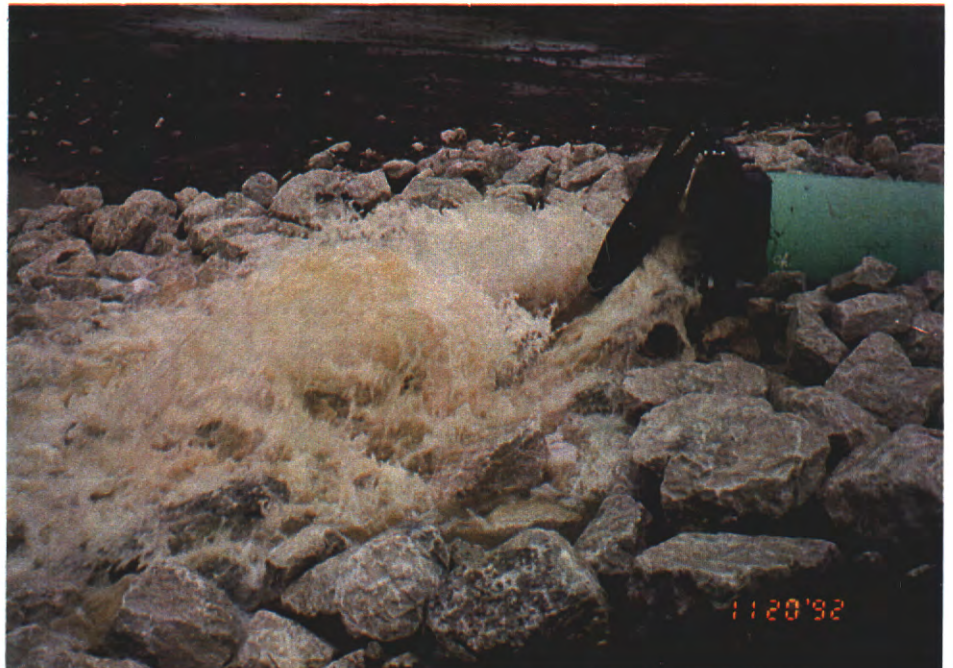
Photo 2. Pump station outfall.
