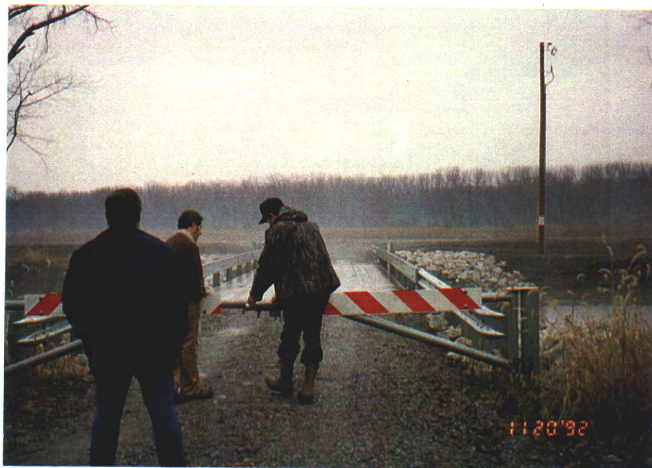
Photo 5. Site access bridge.
