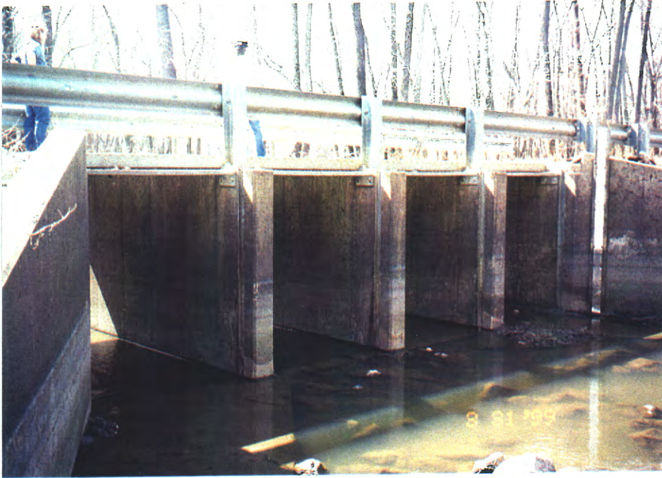
Photo 7. Perimeter water control structure with stop logs removed.
