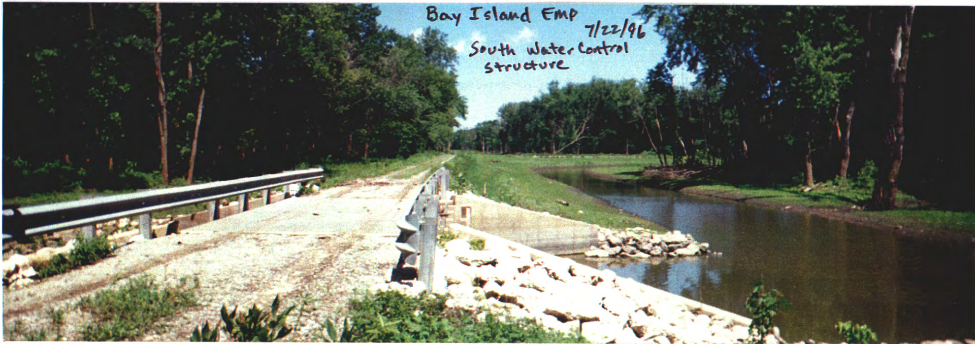
Photo 4. Perimeter levee and south water control structure.
