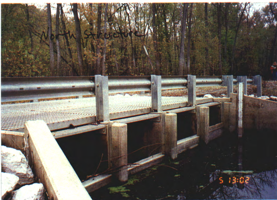
Photo 6. Perimeter water control structure with stop logs in place.
