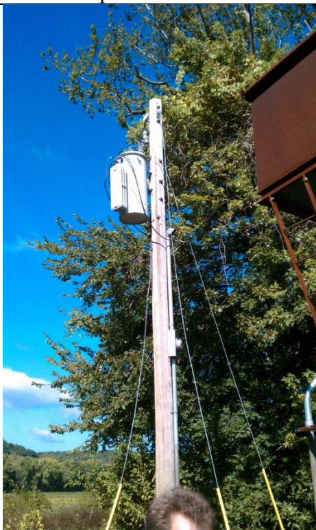
Utility Transformer & Meter Pole
