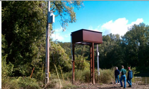
Pump Controller Tower
