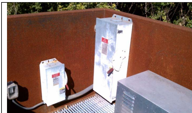
Main Disconnect & Receptacle Transformer
