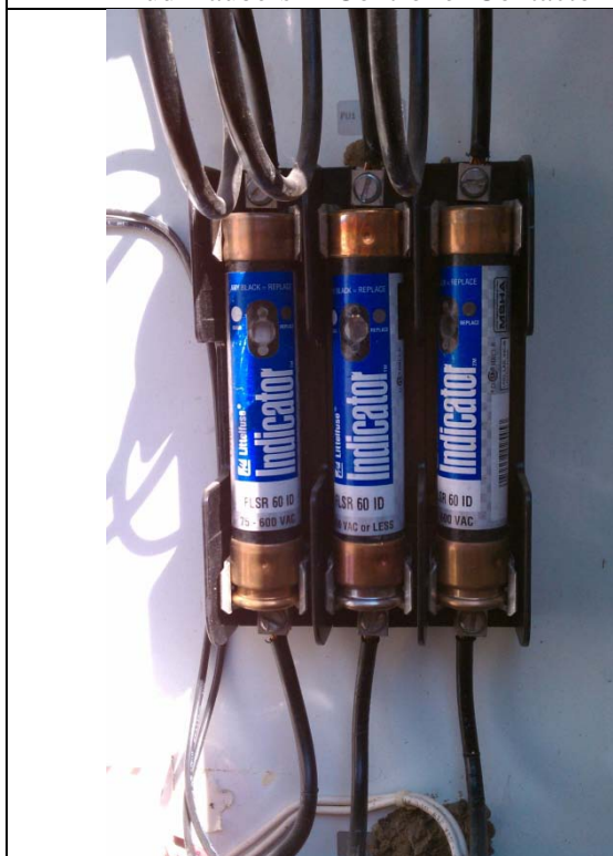
Pump Controller Main Fuses
