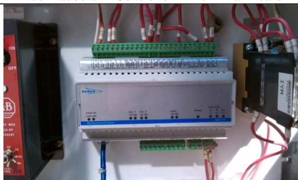
Mud Daubers in Controller in Terminal Board
