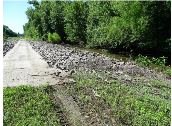
North Spillway riprap in good condition
