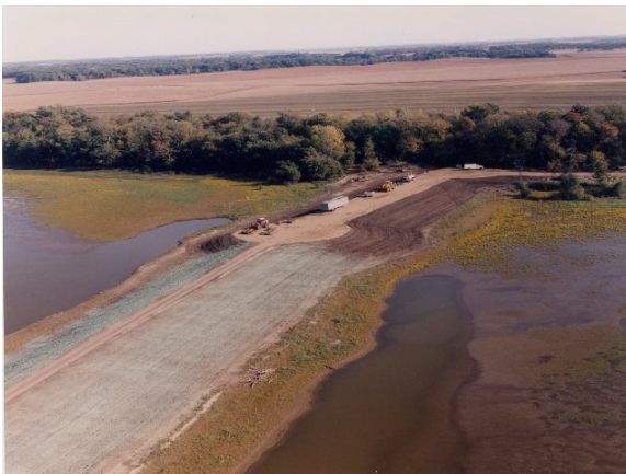
8. Parking area and cross dike under construction. Upper Lake is to the left in photo.
