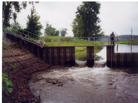
16. Quiver Creek sheet pile dam structure, Sta. 274+60. Constructed by USFWS.
