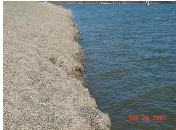
5. North Perimeter Levee. Erosion along waterline.
