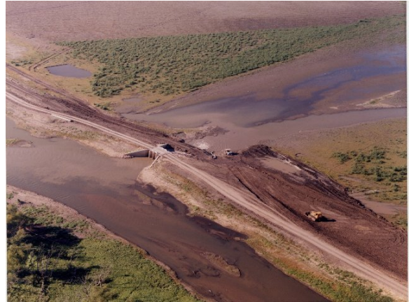
20. Lower Lake levee under construction. New stop log structure at south end of project.
