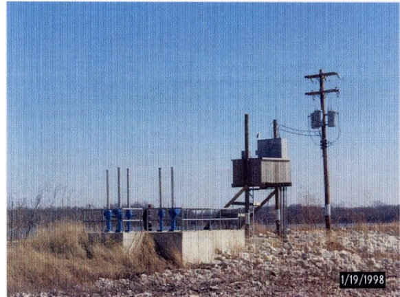
14. Completed 41,000 GPM pump station and electrical platform/transformers.
