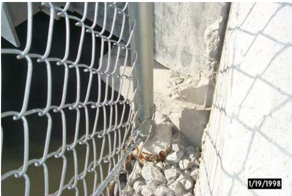
38. Lake Chautauqua. Small crack where abutment overhangs structure. 1 of 2 locations.
