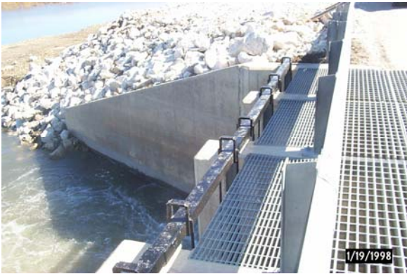
24. Lake Chautauqua. Lower Lake Stop Log Structure. FWS constructed lifting beam for 5 ft wide stop logs.
