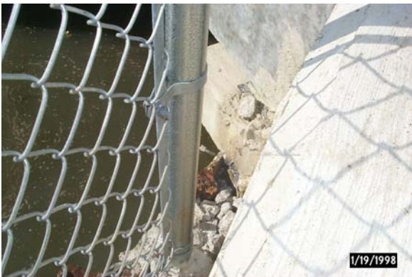
37. Lake Chautauqua. Small crack where abutment overhangs structure. 1 of 2 locations.
