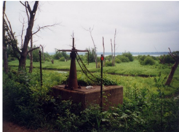
15. 3ft. by 3ft. box culvert and gate from Quiver Creek to Lower Lake. Constructed by USFWS.
