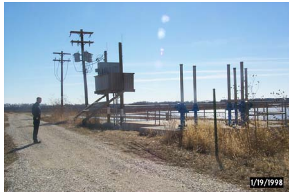
28. Lake Chautauqua. 41,000 GPM pump station and electrical control platform/transformers.
